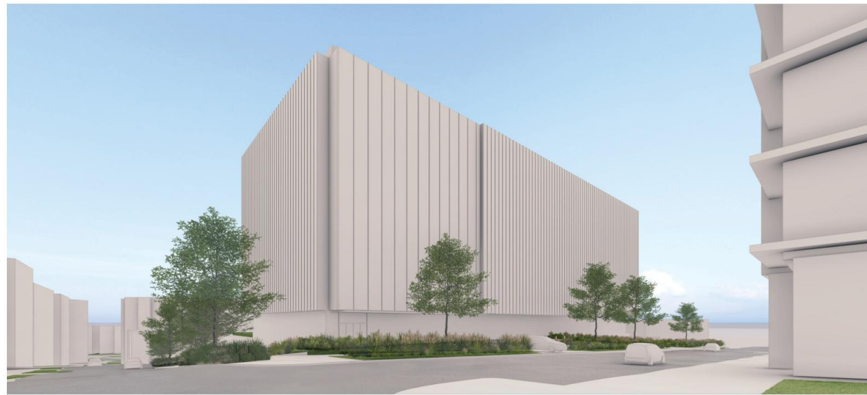
View from the NE Corner
